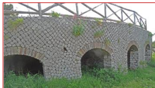
The foundations of the audience chamber at Damecuta
